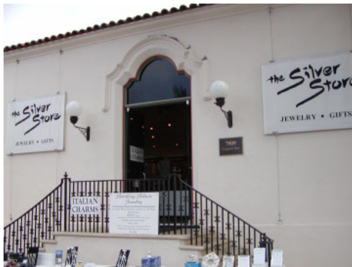
Figure 5 Grand double-staircase entrance to the windowless Art Gallery wing. Taken September 12, 2002.
